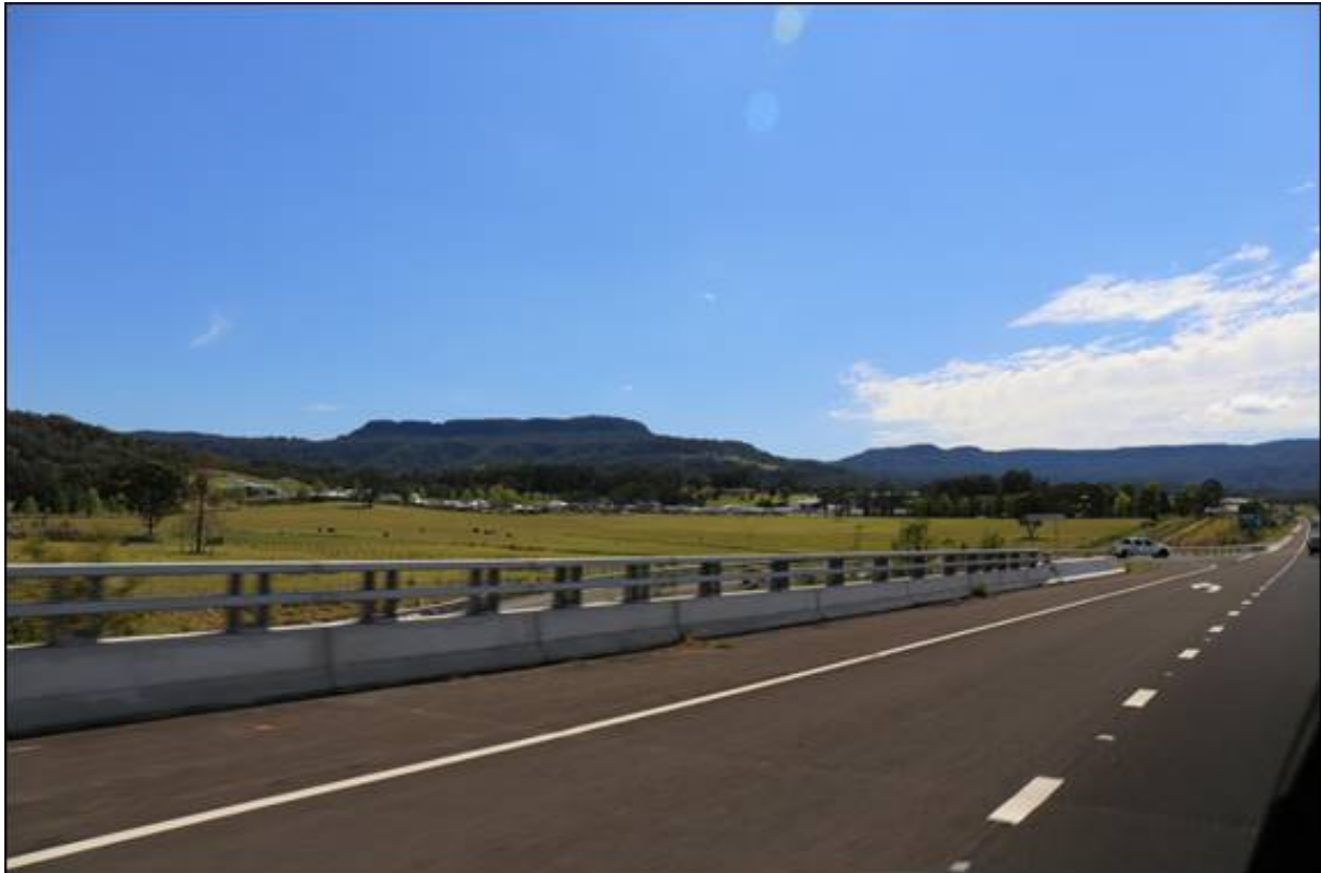
Figure 2: Existing view north toward the subject land from the Princes Highway (Peter Andrews & Associates, May 2019)
